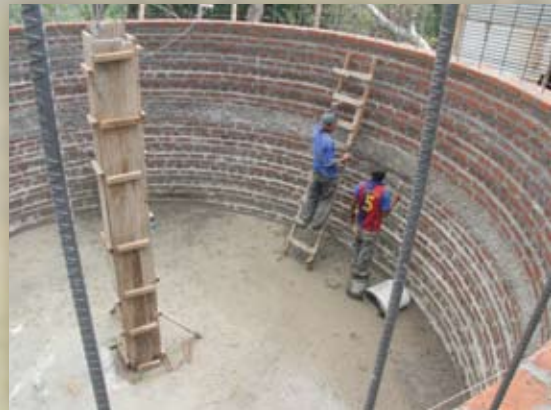
Holding tank under construction for Las Delicias water system.
